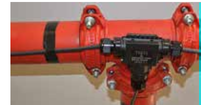
Connection of heating cables (France). Series TH211.
